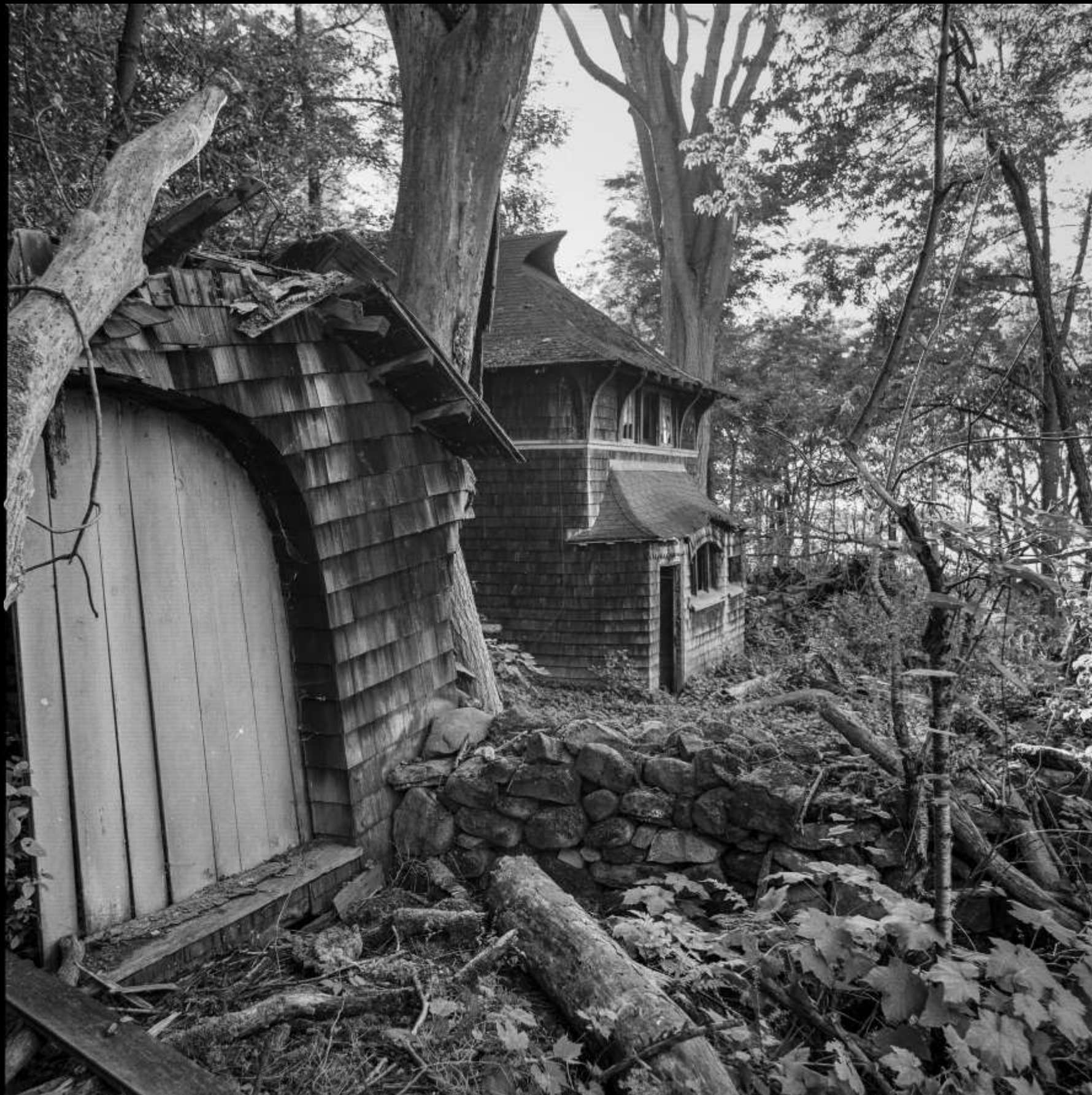
..and at last, the 'Squash Court' building
