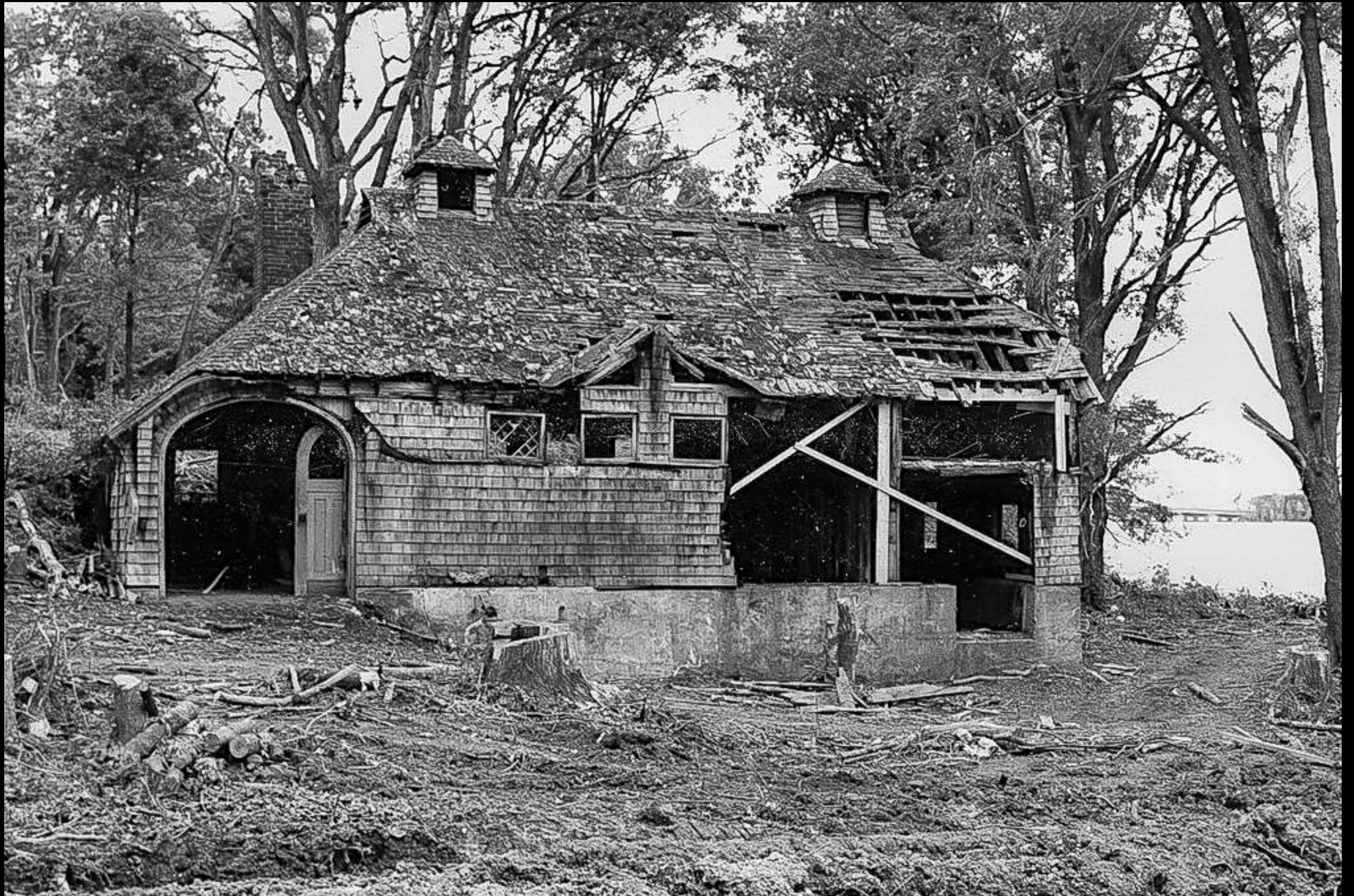
We called this little gem by the water the 'Power House', but it was most likely known as the 'Pump House' in its day.
