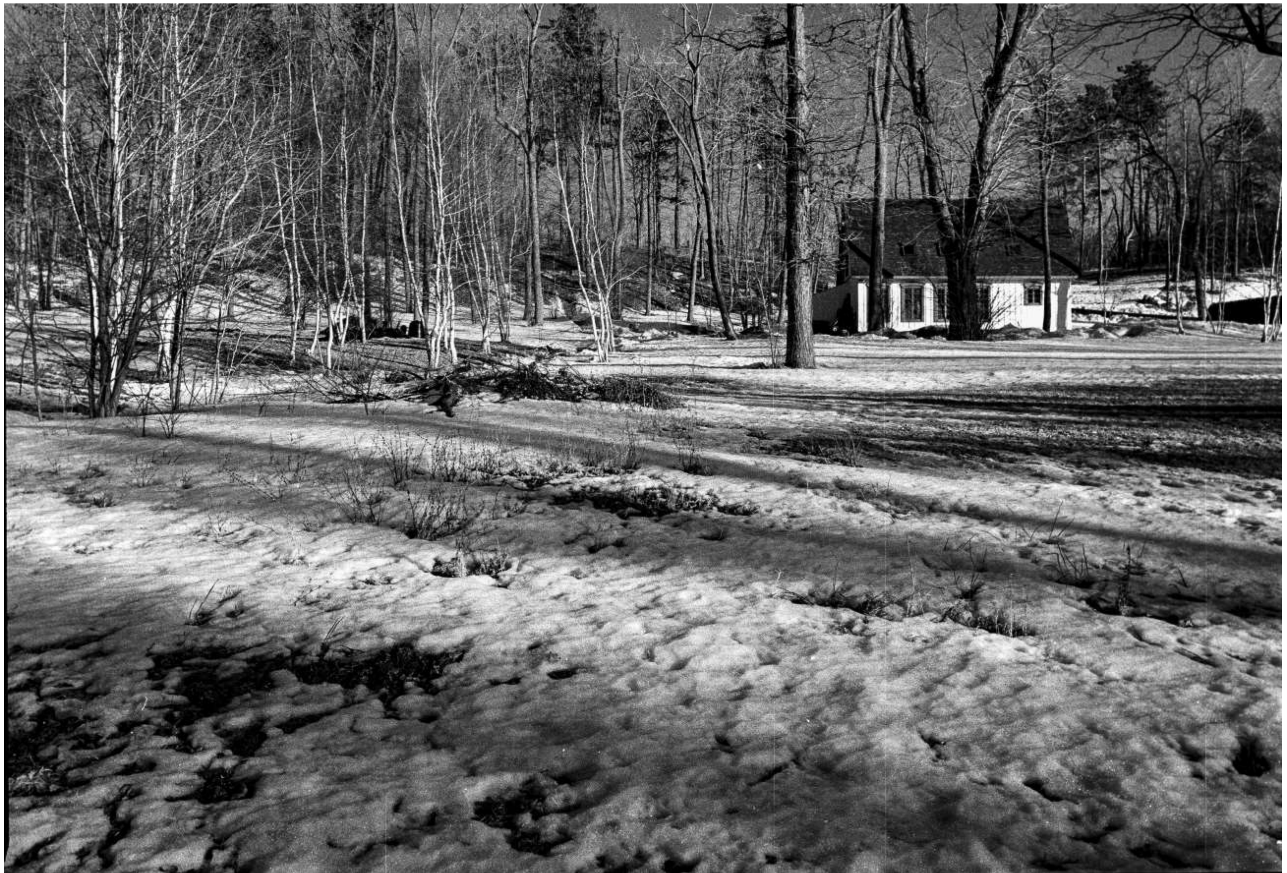
This shows the finished 'White House' and some of the large number of birch trees that were planted at the end of the project
