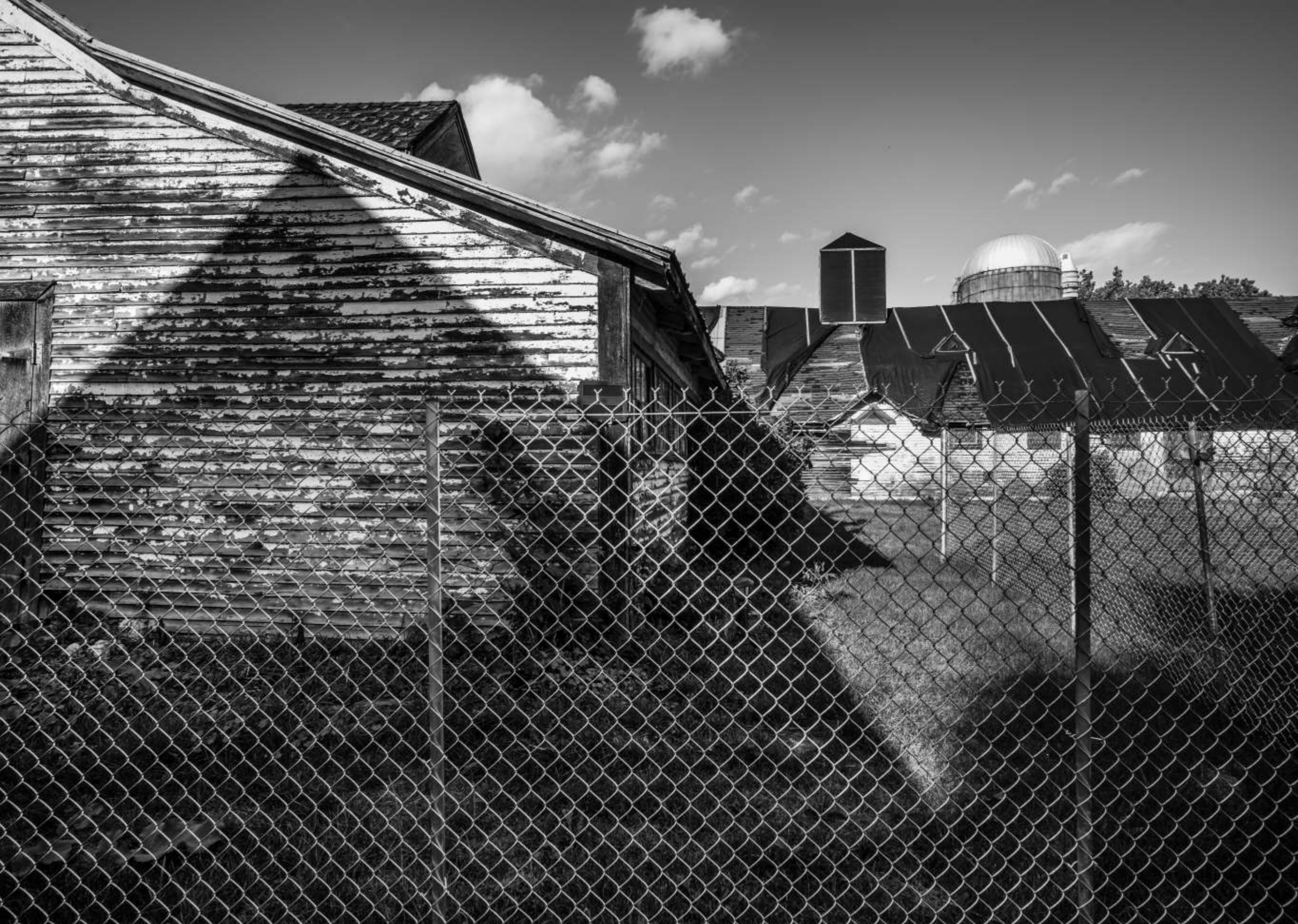
The Maxwell addition joins the original (shown at the rear) and continues to the front
