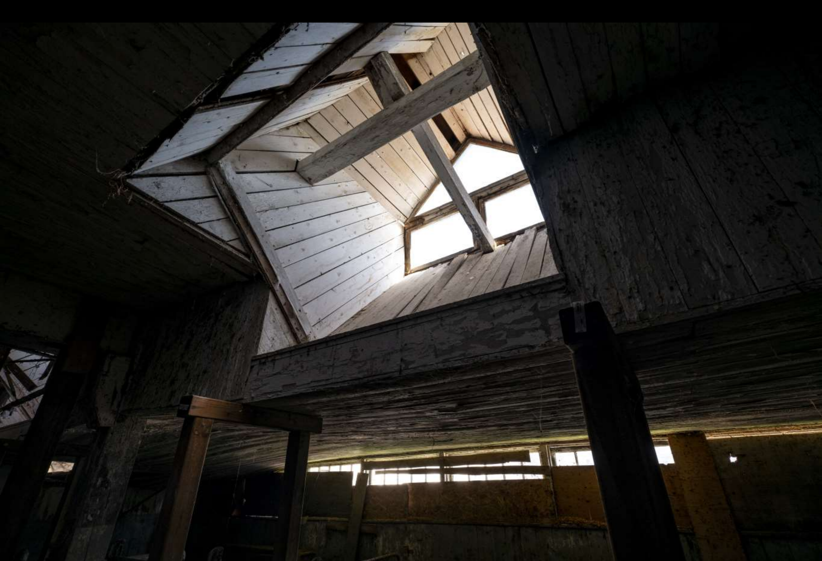
An interesting window detail from the original horse barn that was designed to reflect light downwards into the stable.
