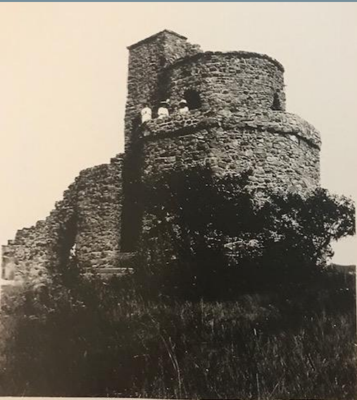
Water tower - Graystones
